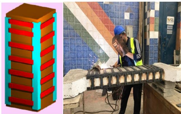
Figure 7: Welding horizontal plates.
