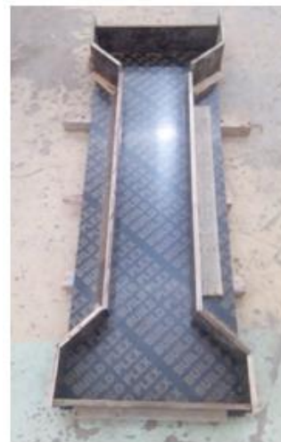
Figure 3: Columns wooden molds.
