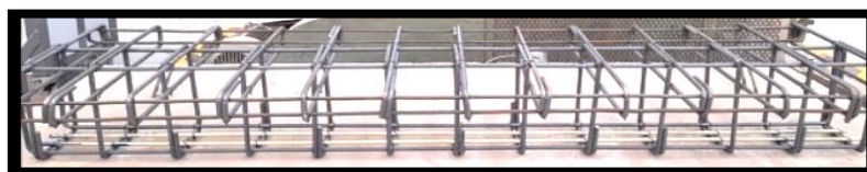
Fig. 3: Beam longitudinal reinforcement
