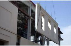
Fig. 3. Prefabricated linear walls [17]
