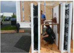
Fig. 7. Insulated Concrete Formwork (ICF [12]
