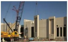
Fig. 4. Prefabricated units [16]
