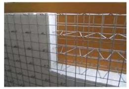
Fig. 8. EPS core panel detail [13]
