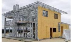
Fig. 5. Lightweight metal structures sample. [18]
