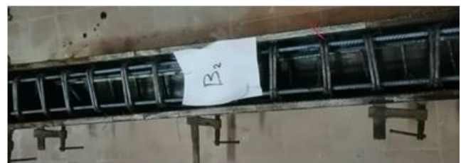
Fig 2. Wooden form and reinforcement of the concrete beams
